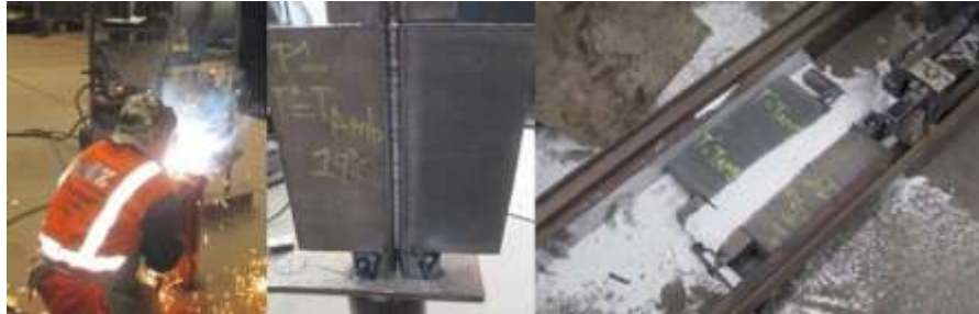
Figure 4. SAW filler welding process according to WPS
