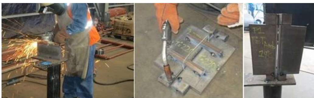
Figure 3. P460NL1 steel plate shoring, double V joint, by FCAW
